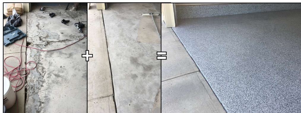
Repair for Coatings
